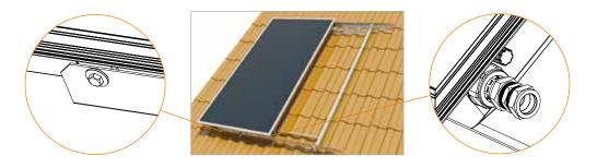
7. Join the second collector and tighten the unions\*. Tighten all screws on the base.
